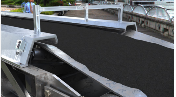
Checking the processing temperature when loading asphalt with thermoMETER UC
